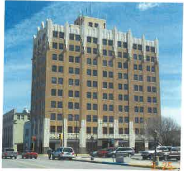
United Life Building, 119 W. Iron Avenue
