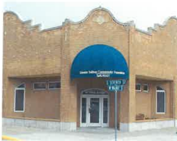
Awning accentuates the main entrance to a building.
