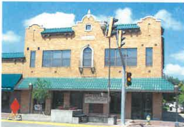
This awning utilizes material compatible with its exterior, Spanish Tile.
