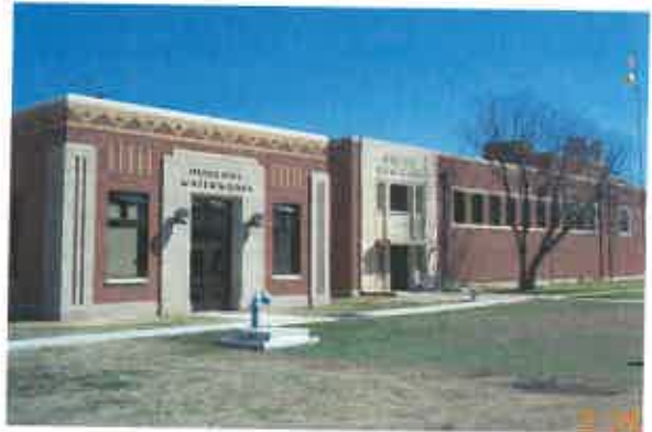
City Water Treatment Plant, 401 S. 5th Street
