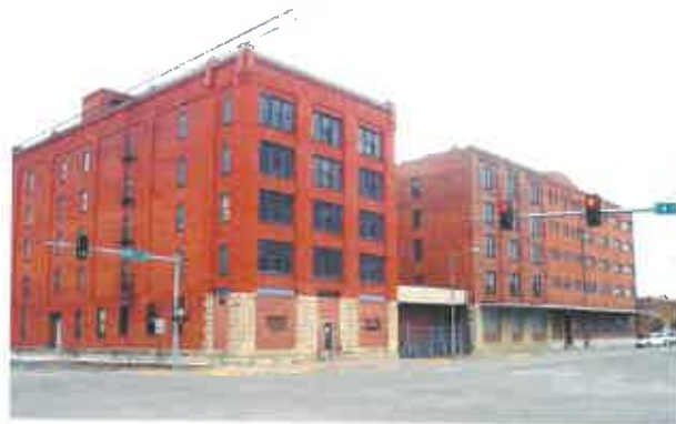
248-254 N. Santa Fe Avenue, H.D. Lee Complex
